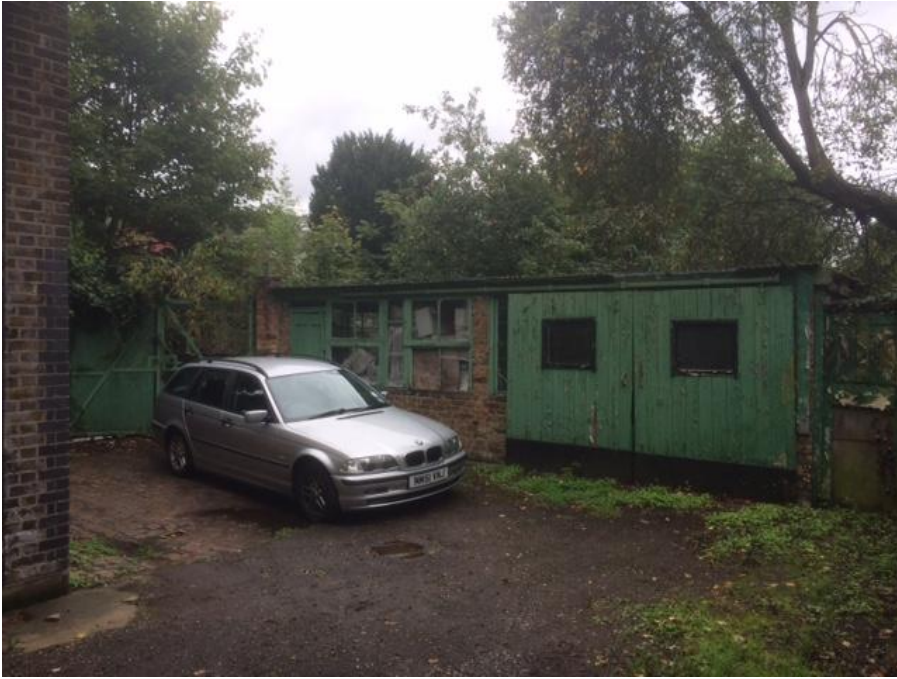
Site visit photo – existing garage building
