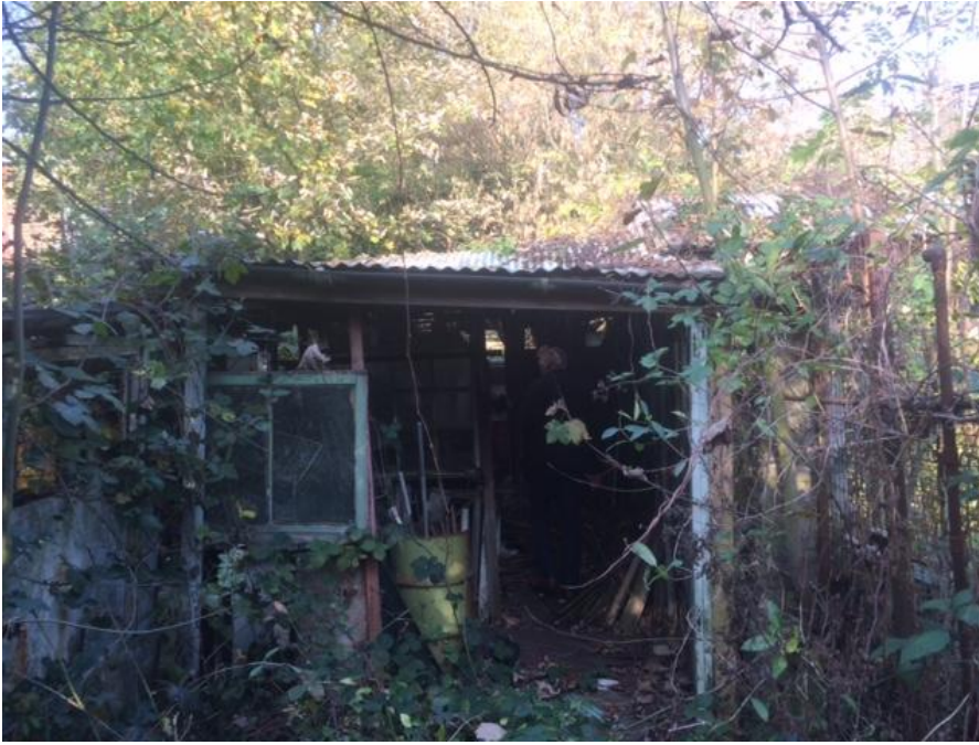
Site visit photo - existing structure on site (looking west)
